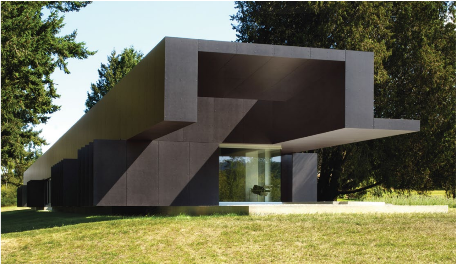
Linear House, Salt Spring Island, British Columbia (Picture: James Dow and Patkau Architects)
